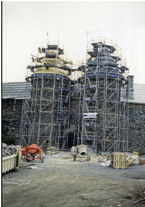
Restoration of the tower roofs
