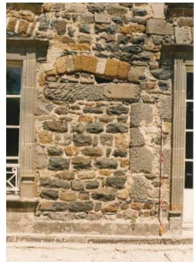
Inner court facade
