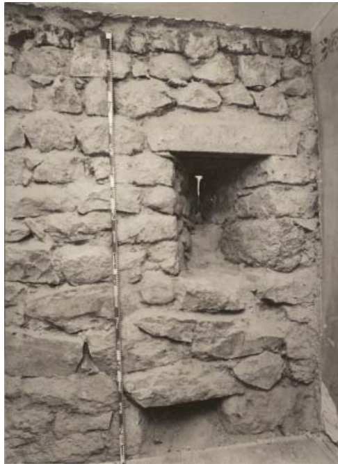
Shooting slit north wall linking bay from inside
