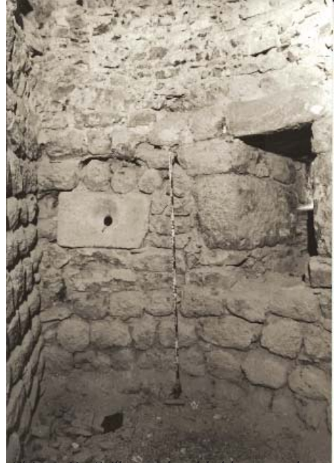
Château Du Sailhant -- hand-held cannon shooting slit added to west entrance tower. (Photograph by Sélysette Somorjay)
