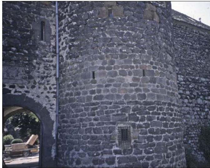
West entrance tower with shooting slits added in the 16th century (Photograph by Author)
