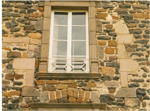
Inner court facade vestiges of arched opening to granary
