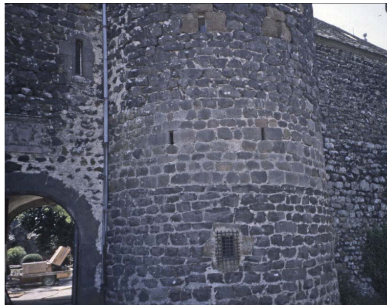
West entrance tower with shooting slits added in the 16th century (Photograph by Author)
