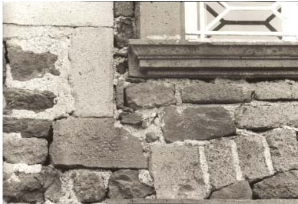
Curb stone in vestige of arched opening to granary
