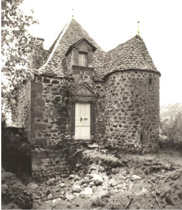
Donjon with moat partially excavated
