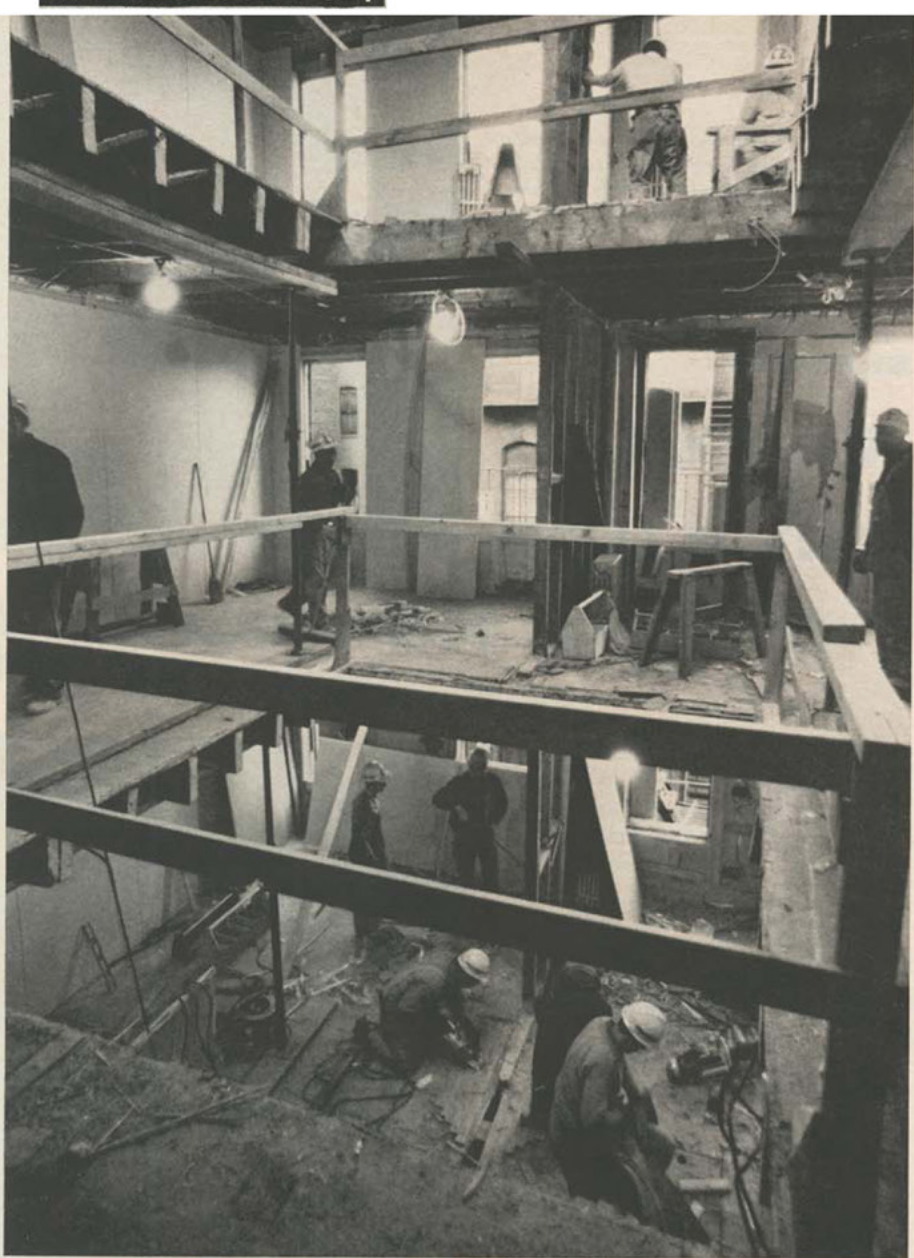
While supervisor with walkie-talkie directs crane on street below, preassembled "cores" of kitchen and bathroom units are lowered through a shaft cut into the building's floors.
